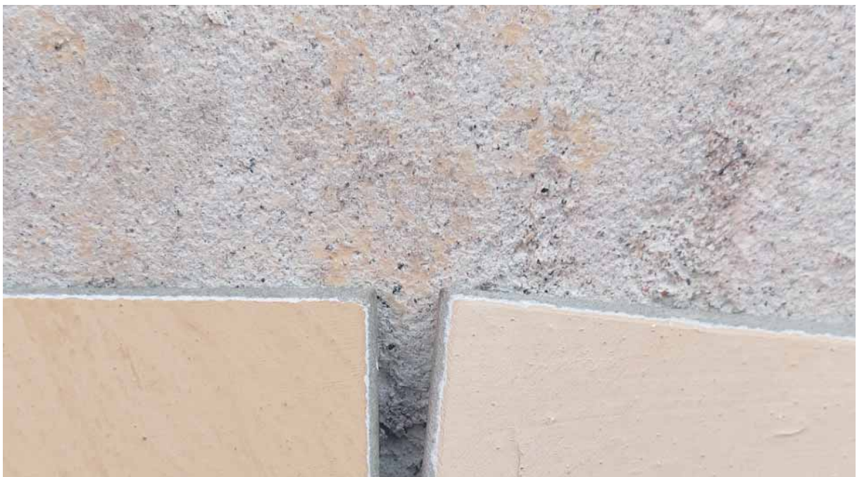
Ljusare kulörer under befintlig puts.
